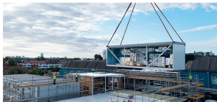
Prefabricated process modules are manufactured, transported, and installed with high precision, an approach that shortens project timelines and minimizes disruption at the customer's facility. Photo: KeyPlants.
