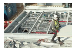
These photos show assembly of a modular facility by KeyPlants
