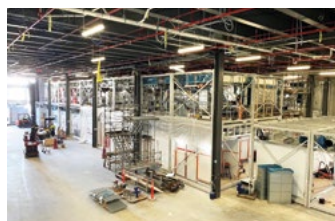
Internal Modules "Box-in-Box"
